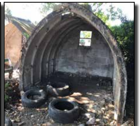
Left: The last remaining half arch of a Stanton Shelter at Fairfield, Westhumble. Above: A slightly more complete example of a Stanton Shelter.
